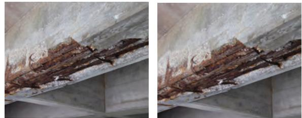
In addition, the onset of steel corrosion in concrete may be accelerated by chlorides that can enter the concrete from the batching/mixing process, deicing chemicals, and/or the environment. Anodic Ring Phenomena, also known as the “Halo Effect,” is a special form of metal corrosion in which “new” corrosion sites develop immediately around repair areas.
